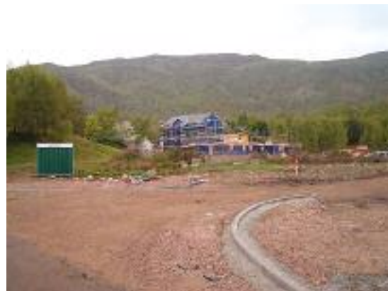
Fig. 3 - Staff Block under Construction
