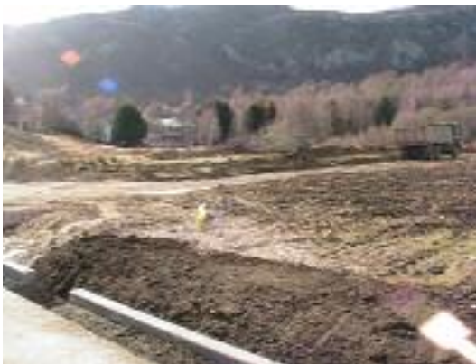
Fig. 2 - View of Site from North East
